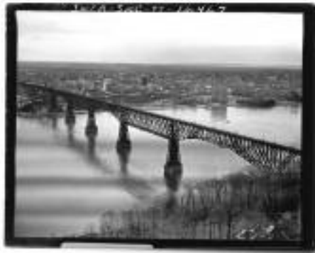
The Poughkeepsie-Highland Railroad bridge in 1978 and, top, on October 4, 2009 when it opened as a Mid-Hudson trail link for walkers and bikers.
