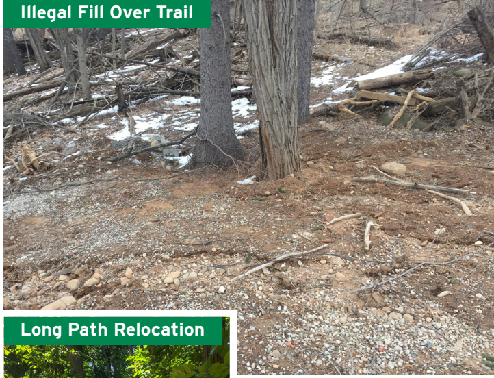
Illegal Fill Over Trail
