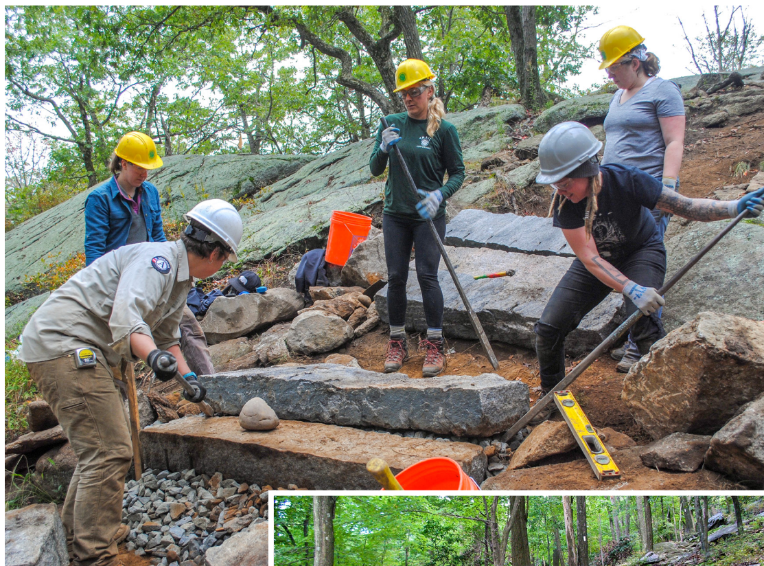
Before the start of the Bear Mountain Trails Project, the Appalachian Trail on Bear Mountain was as wide as 40 feet in some places (right). To accommodate the high volume of visitors, the sustainable solution was to build stone steps up the majority of the mountain (above).
