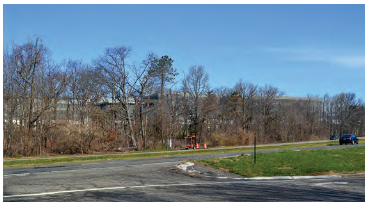
The Trail Conference played an important role in LG Electronics USA amending the planned height of its new headquarters in Englewood Cliffs, N.J., protecting the viewshed along the Palisades. Read more on pages 4-5.
