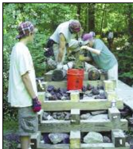
From piling construction...
