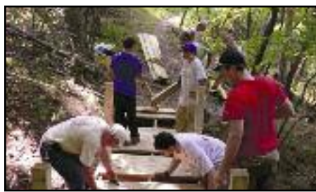
Top to bottom: Eagle Scout candidate John Quartucio's finished bridge on George's Island; getting ready to float the bridge from the mainland; putting the bridge into position; placing the decking.
